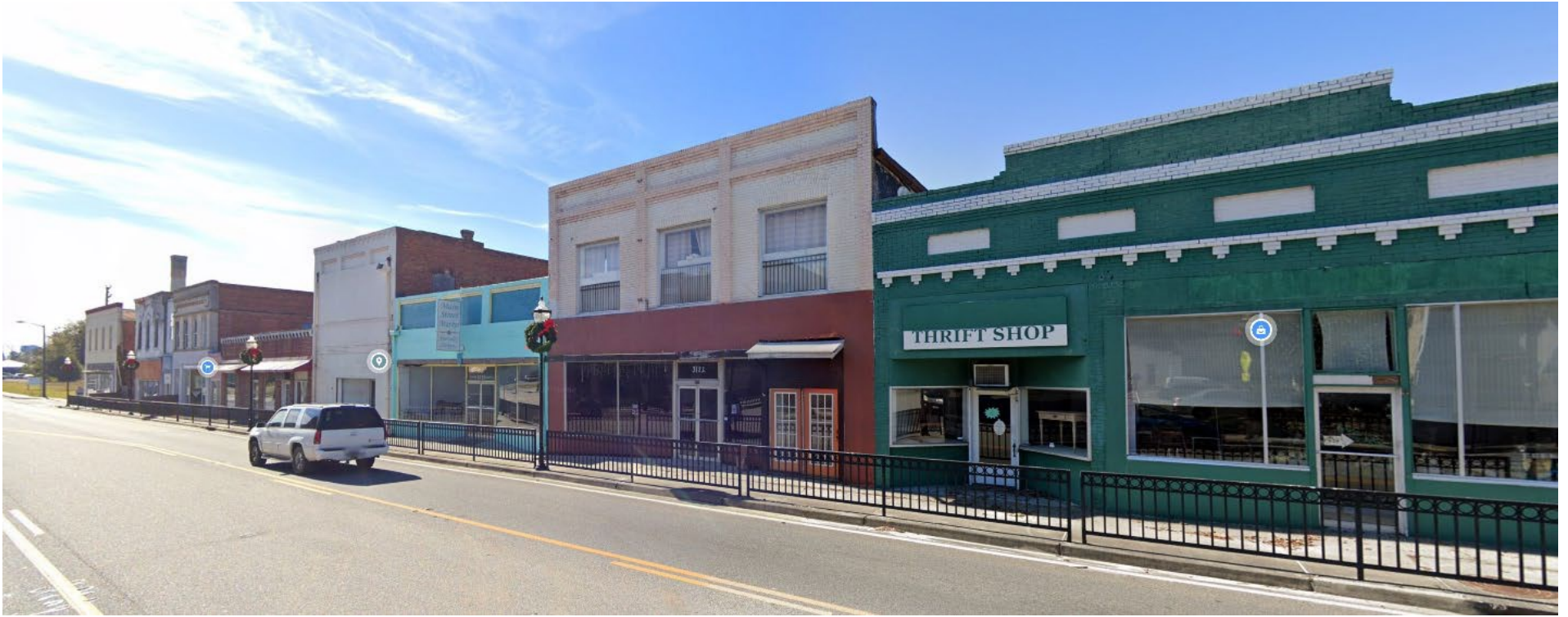
Bamberg, SC. Example shows aesthetic variation to avoid monotony and overly linear facades.
